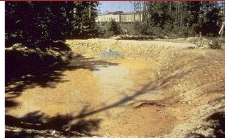
Sediment basins are used to trap sediments and temporarily detain runoff on larger construction sites.
